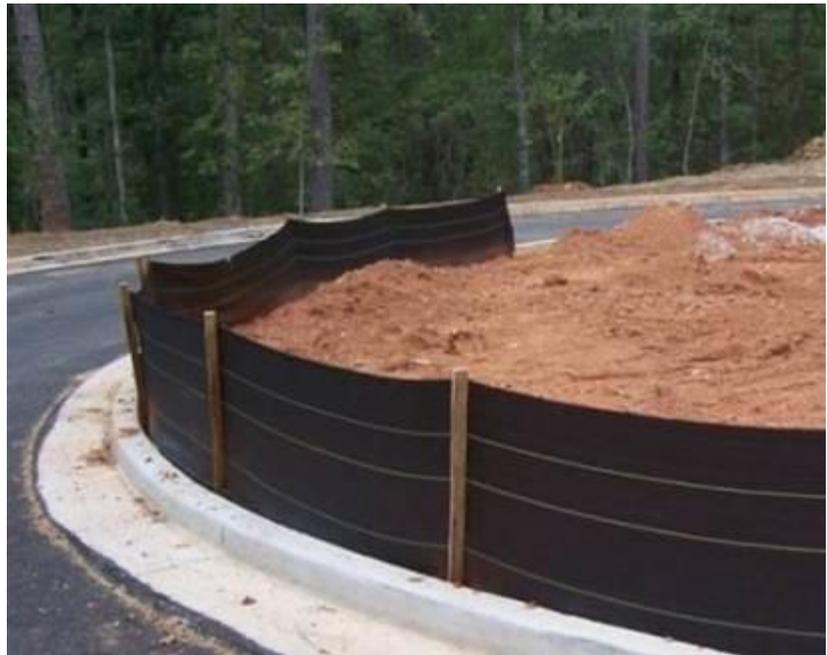
*A silt fence on a construction site retains soil that might otherwise be washed into bodies of water. Although silt fences are quite common on transportation construction sites, the effectiveness of a silt fence as an environmental mitigation measure depends upon its proper installation and maintenance during construction activities.*
