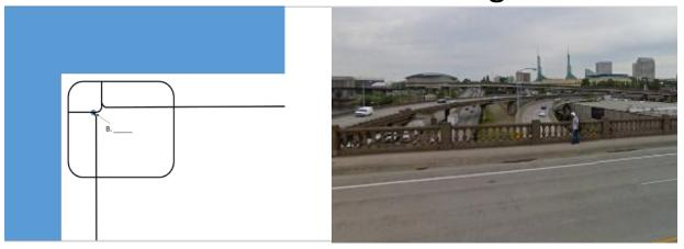
Description: This particular bottleneck occurs on one of the central y interchanges. Where the two branch segments merge, there is inadequate space for vehicles to converge onto the root segment causing congestion and many crashes. The probe data represents the root segment.
