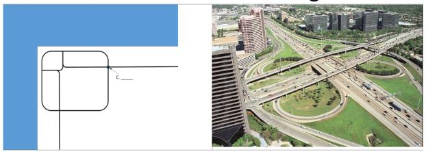
Description: The interchange between the Factiuousville Beltway and the freeway that goes towards the eastern suburbs and exurbs is currently configured as a cloverleaf interchange. Due to the growth in the immediate vicinity of the interchange, traffic can get heavy at the low capacity interchange. The probe data shown is representive of a freeway segment just before the interchange.
