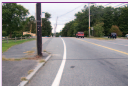
Vertical curve in roadway at RSA location. IMAGE COURTESY of Town of Tiverton, RI.
