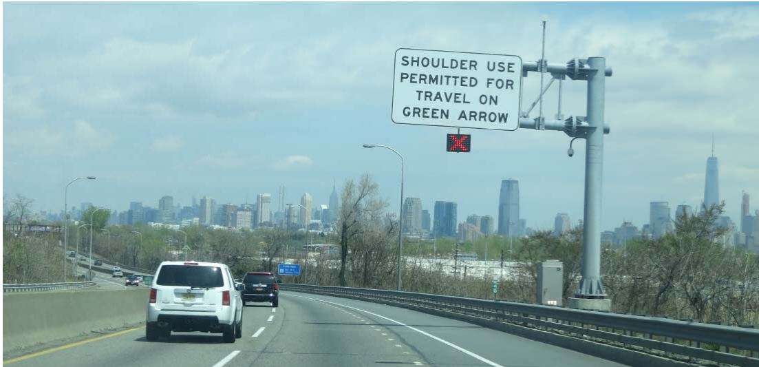
Figure 59. Photo. Mast Arm Dynamic Lane Control Sign, New Jersey Turnpike Newark Bay Extension. (Source: Kittelson & Associates, Inc.)
