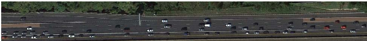
Figure 71. Photo. Off-ramp striping, I-66.
