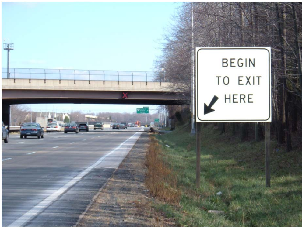
Figure 63. Photo. Static signage denoting permitted use of shoulder to exit during non-operational hours of shoulder use, I-66 mainline.
