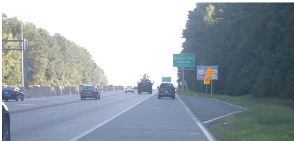
Figure 36. Photo. Emergency Turnout, Georgia. (Source: Georgia Department of Transportation)
