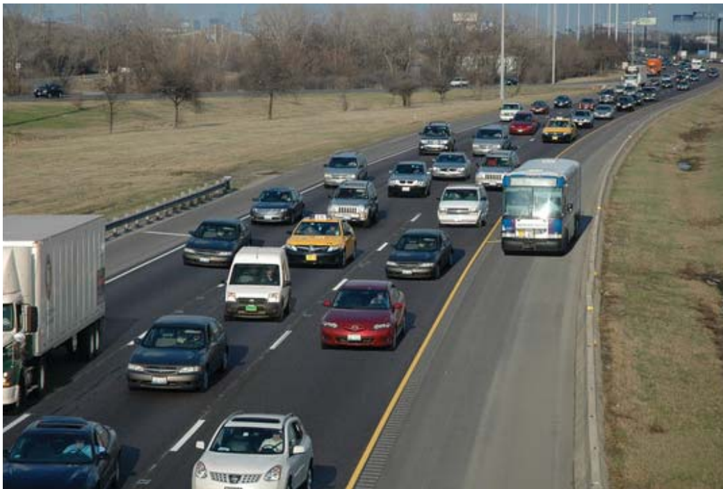
Figure 3. Photo. Bus-on-shoulder operations on the left-shoulder in Chicago. (Source: Pace Bus)
