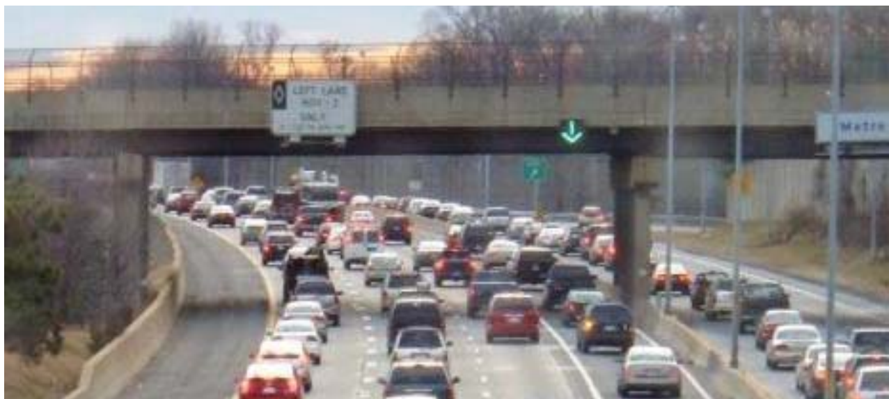
Figure 5. Photo. Previous Static Part-time shoulder use on I-66 in Northern Virginia (Source: Virginia Department of Transportation)
