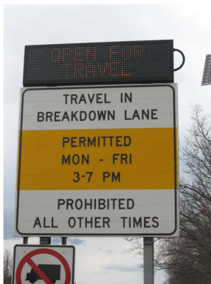
Figure 57. Photo. Dynamic sign signifying the shoulder is open for use, I-95 breakdown lanes.
