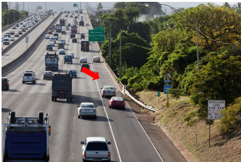
Figure 66. Photo. Edge lines and “shldr lane” work markings on a part-time shoulder use section of I-H-1.
