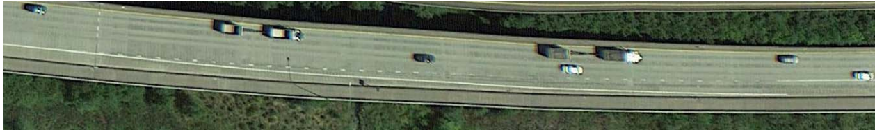
Figure 67. Photo. Edge line markings at the start of part-time shoulder use segment, US 2. (Source: Google Earth)
