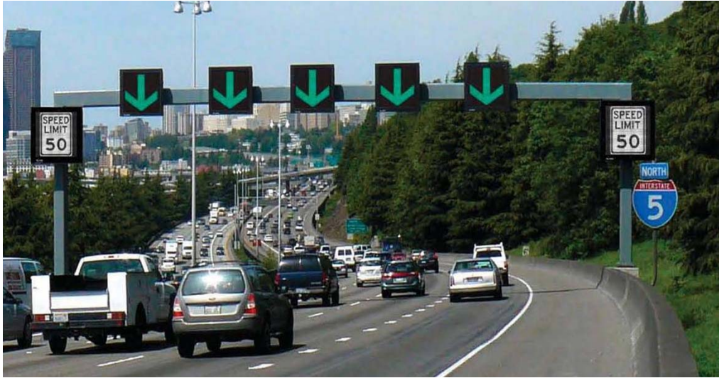
Figure 38. Photo and Illustration. Example of full gantry ATM deployment in Washington State (no part-time shoulder use).
