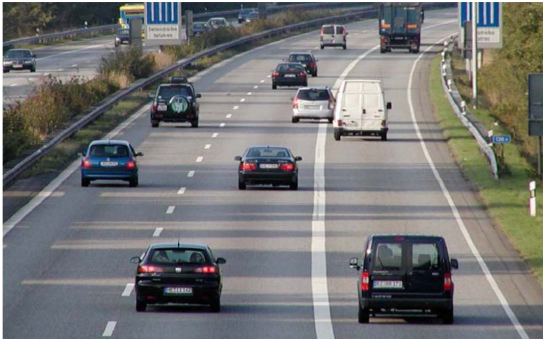
Figure 7. Photo. Part-time shoulder use in Germany.
