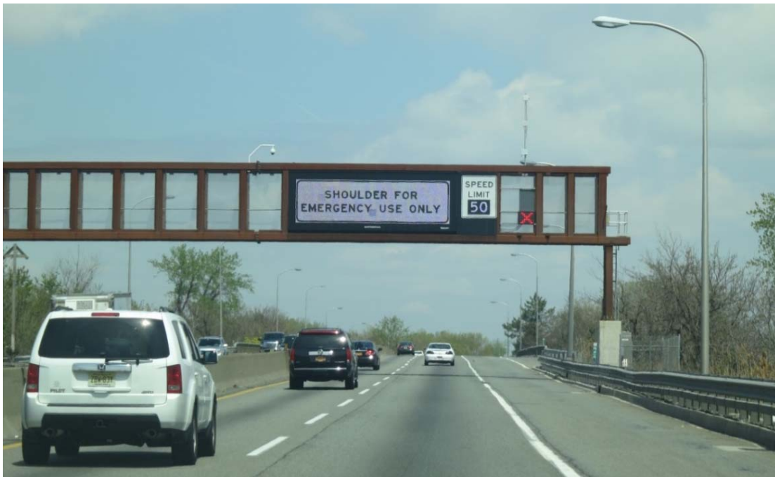
Figure 60. Photo. Dynamic Lane Control Sign on Gantry, New Jersey Turnpike Newark Bay Extension. (Source: Kittelson & Associates, Inc.)
