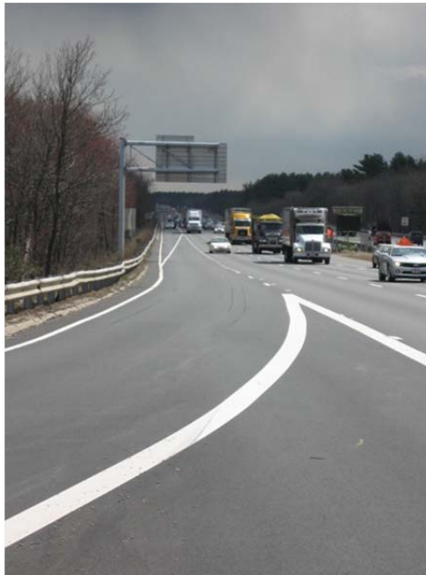
Figure 70. Photo. Off-ramp striping, I-93.
