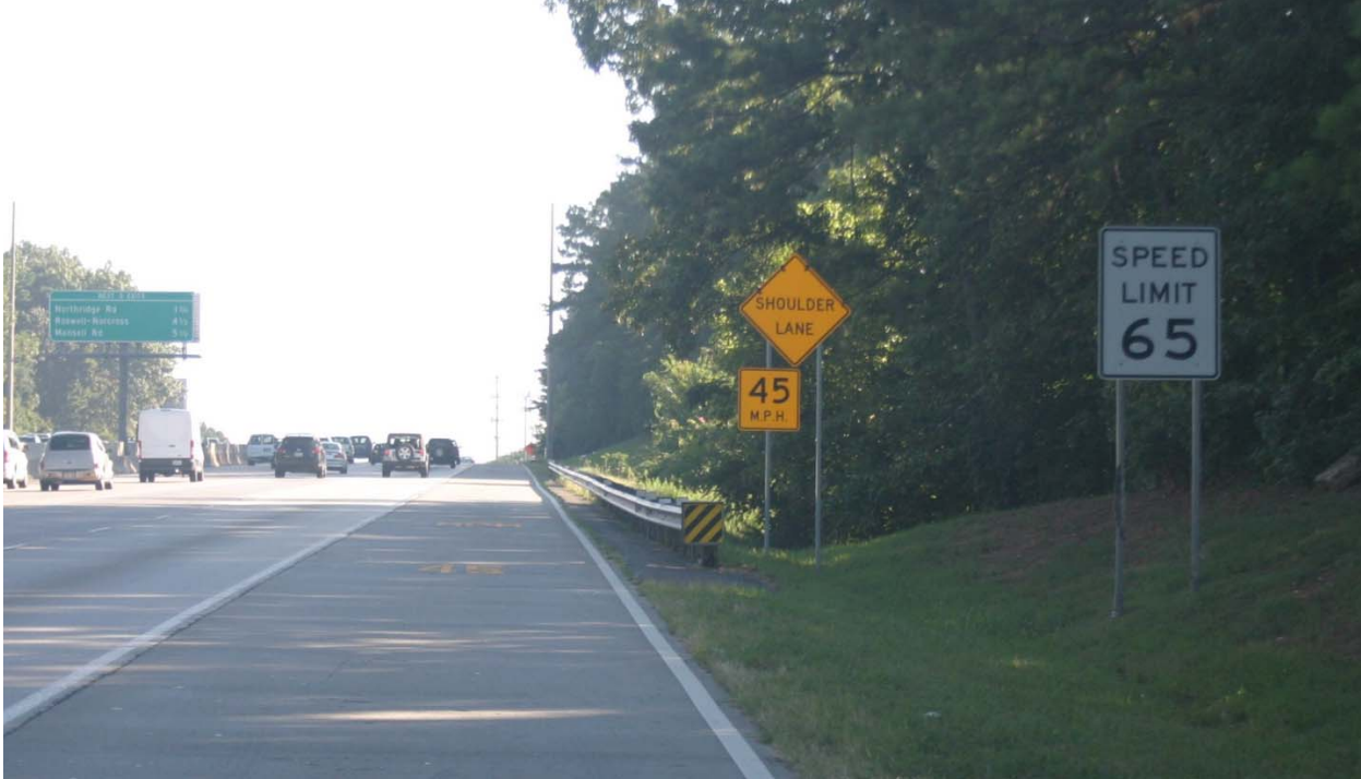
Figure 49. Photo. Warning sign along part-time shoulder use segment, GA 400. (Source: Georgia Department of Transportation)
