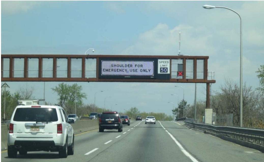
Figure 6. Photo. Static part-time shoulder use on New Jersey Turnpike Newark Bay Extension with variable speed limit and changeable message sign.
