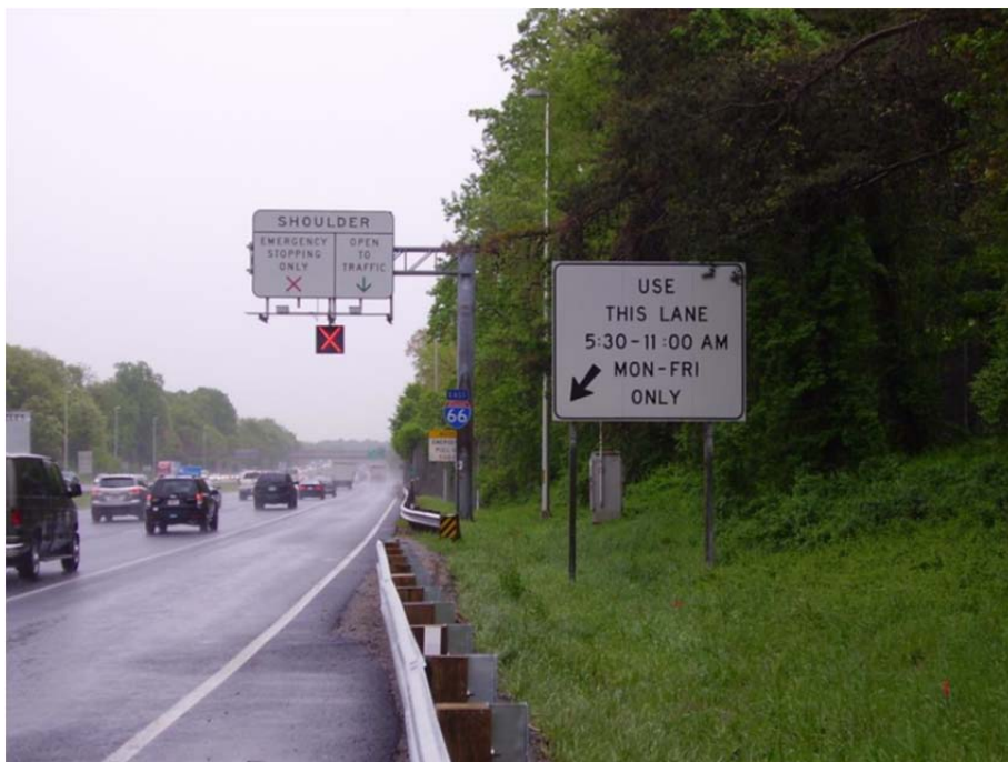
Figure 61. Photo. Combination of static and dynamic signage, I-66 mainline. (Source: Virginia Department of Transportation)
