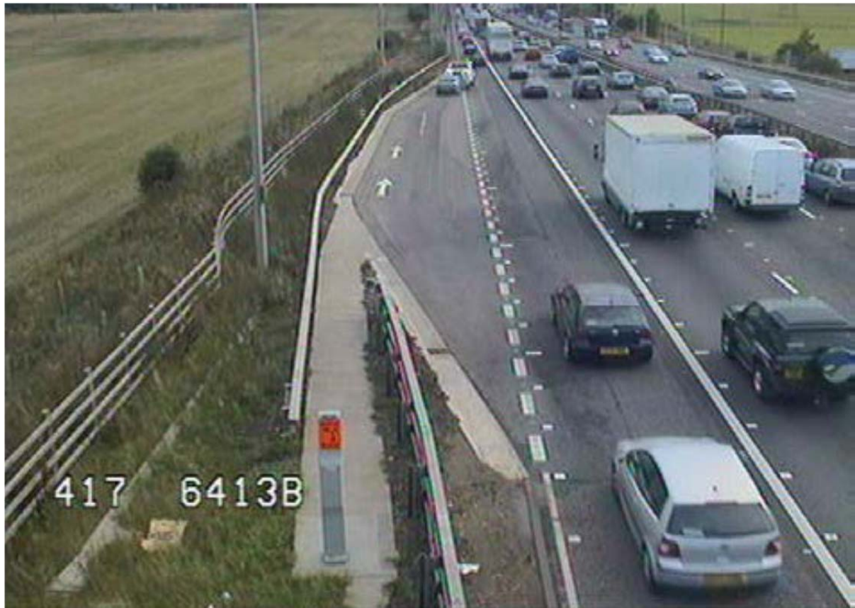
Figure 35. Photo. Emergency Turnout, UK. (Source: FHWA ATM Screening Guidelines)
