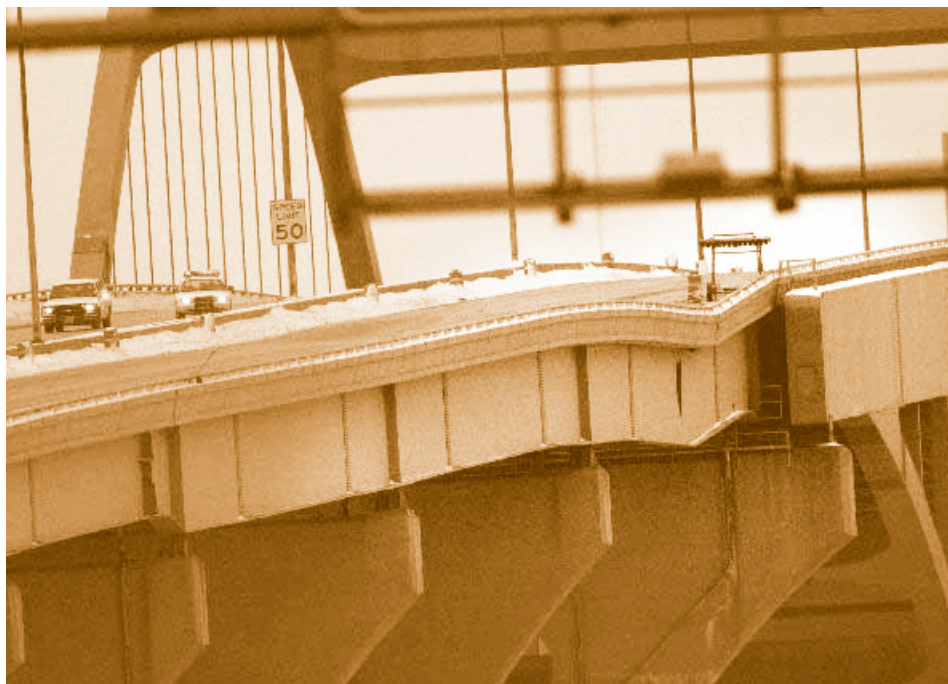
Figure 31 Structural failure on Daniel Webster Hoan Memorial Bridge, December 13, 2000.
