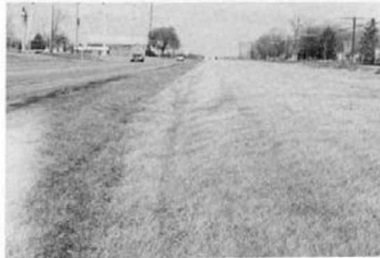
Rural roadside hazard rating of 1.
