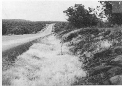
Rural roadside hazard rating of 3.
