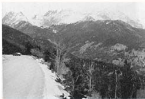
Rural roadside hazard rating of 7.
