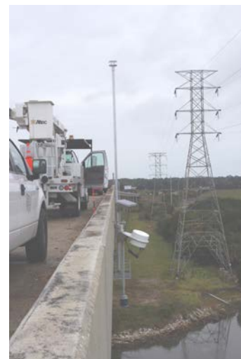
Figure FL-1. FDOT bridge wind speed monitor installation.
