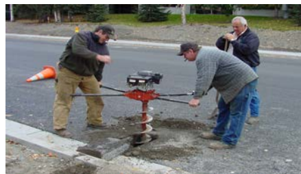
Figure AK-2. Boring hole for temperature probe.
