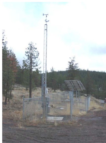
Figure CA-2. Road weather information system at Fredonyer East ICWSs.
