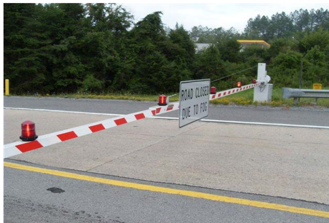
Figure TN-4. Swing gate.
