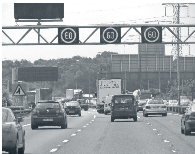
Figure 1. England: variable speed limit in Birmingham (vehicles enter the roadway from the left, opposing traffic is on the right, and speeds shown are in miles per hour).
