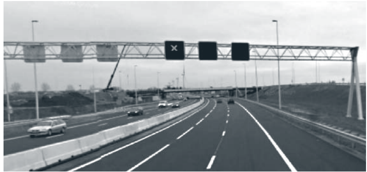
Figure 25. Netherlands: A12 plus lane closed to traffic. (5) SOURCE: GOOGLE EARTH™
