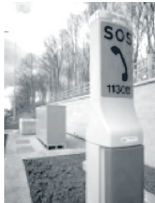
Figure 40. England: telephone in an emergency refuge area. (19)
