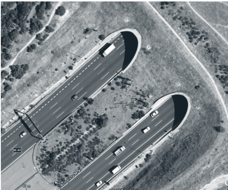
Figure 11. Spain: view of approach and exit from tunnel. (5)
