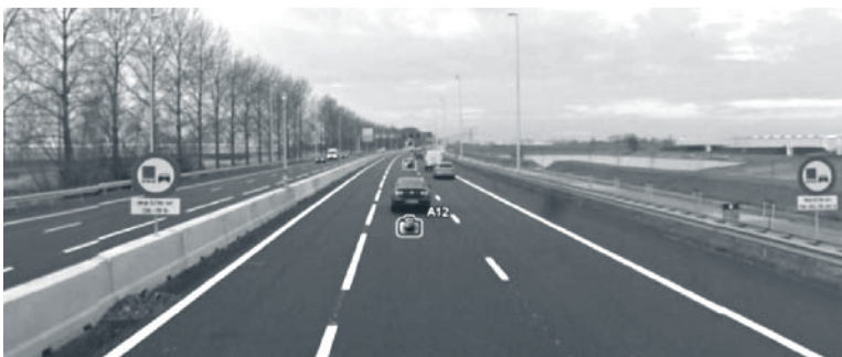
Figure 24. Netherlands: A12 plus lane with current plus lane markings and truck restriction. (5)
