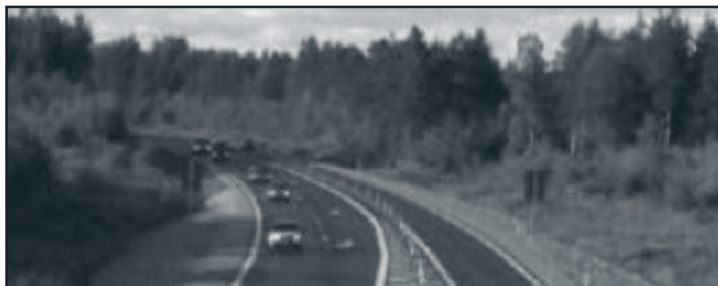
Figure 55. Sweden: typical 2+1 median barrier design on 13-m paved width. (34)
