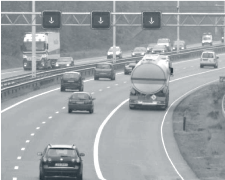
Figure 22. Netherlands: hard shoulder running.
