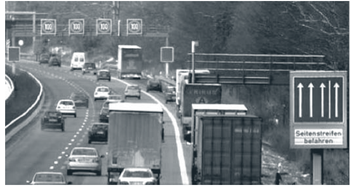
Figure 4. Germany: shoulder use and variable speed limit in Hessen (speeds are in kilometers per hour). (17)
