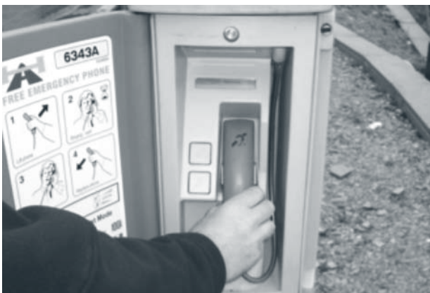
Figure 40. England: telephone in an emergency refuge area. (19)
