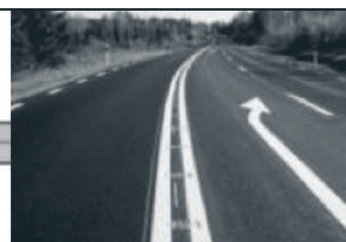
Figure 56. Sweden: overtaking lane principles with rumble or barrier median. (34)
