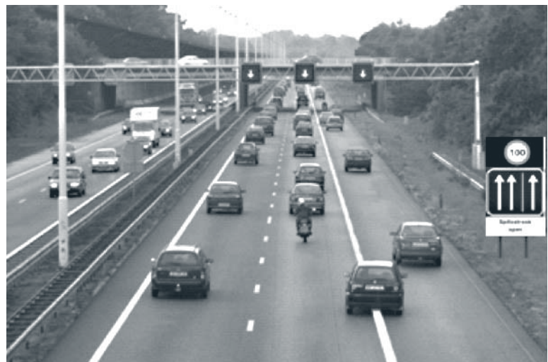
Figure 21. Netherlands: hard shoulder running. (15)
