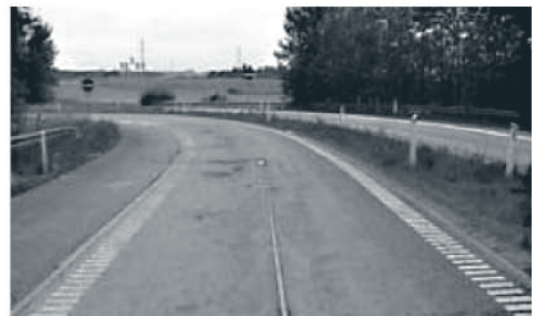
Red flashing lane lights
