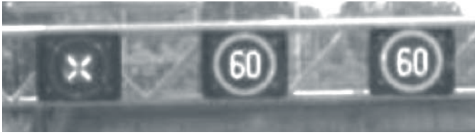
Variable speed limit and shoulder control signs in use (speeds are in miles per hour)
