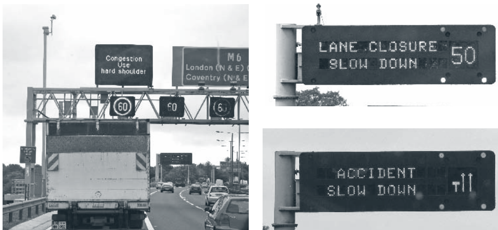
Figure 3. England: variable message signs in Birmingham (vehicles enter the roadway from the left, opposing traffic is on the right, and speeds shown are in miles per hour).
