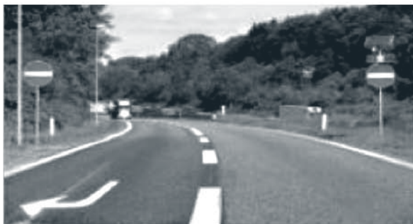
Flashing lights on “No Entry” sign
