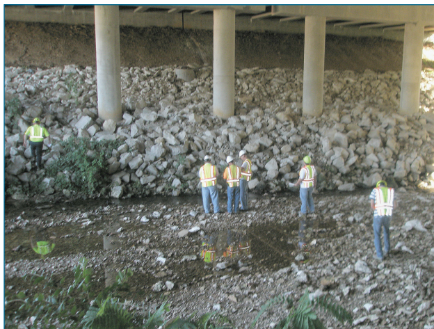
Course participants are inspecting a bridge as part of a field trip. Credit: Douglas Blades, FHWA
