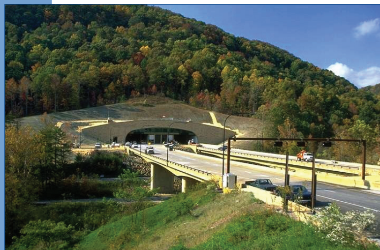
The Cumberland Gap Tunnel is a highway tunnel that carries U.S. Route 25 East under Cumberland Gap National Historical Park between Tennessee and Kentucky. Shown here is the east portal from the Tennessee side.
