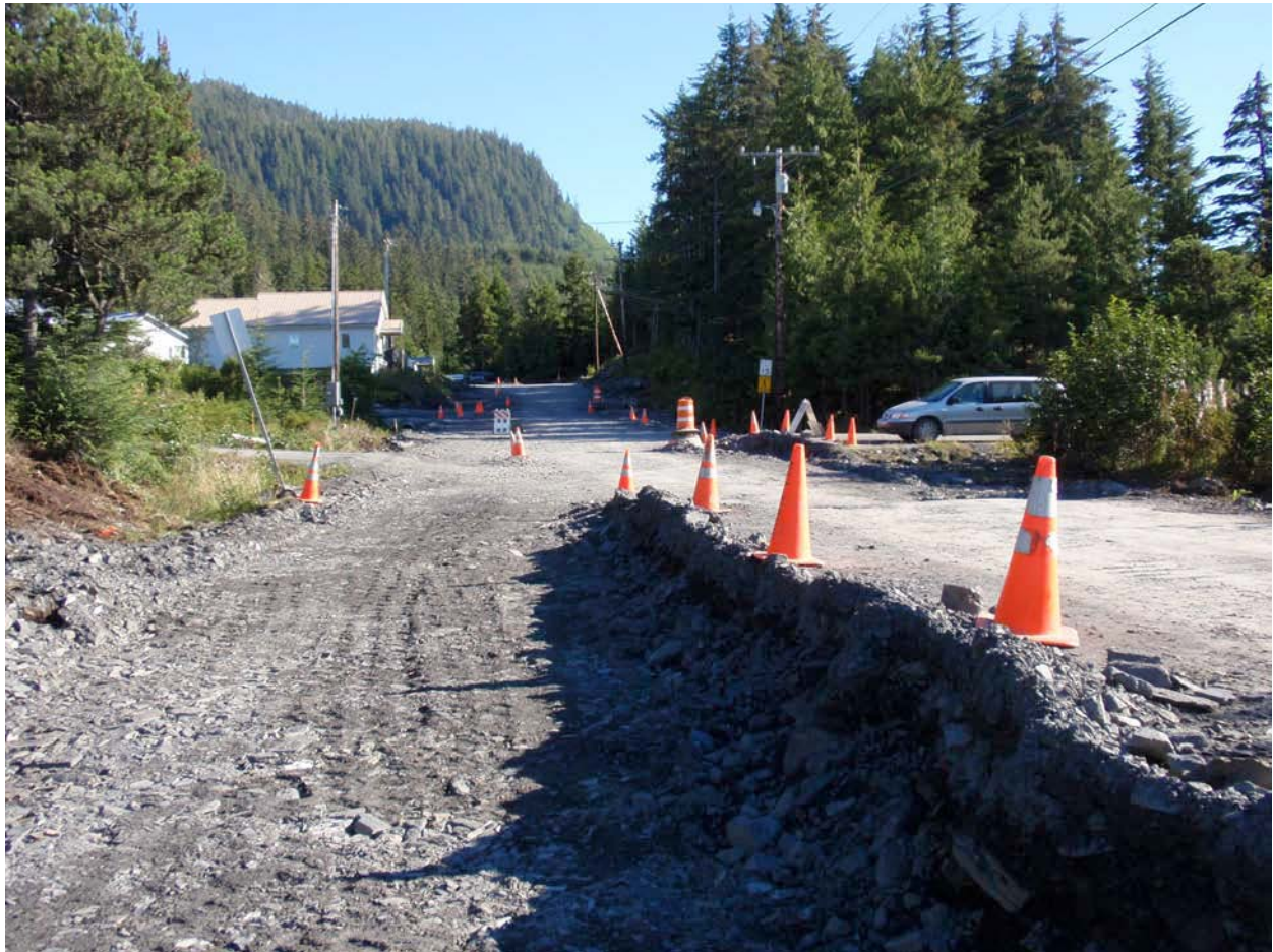
Excavation on Etolin Street
