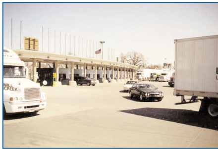
Primary border inspection facility on the U.S. side of the Peace Bridge, Buffalo, NY
