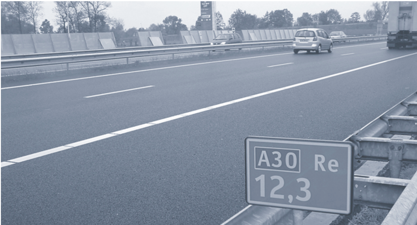
Figure 19. Two-layer porous asphalt section on A28.
