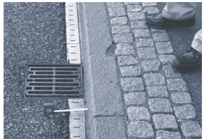
Figure 2. Oster Sogade in Copenhagen with PA8 (8-mm porous asphalt surface).
