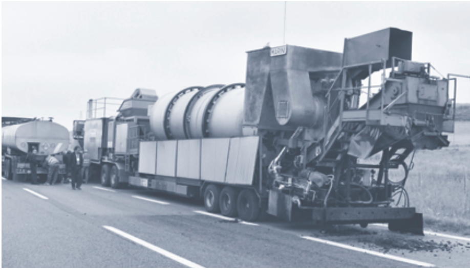
Figure 11. Recycling a porous pavement in Italy.
