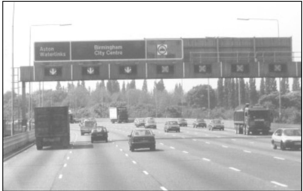
Lane control signals on freeway in England.
