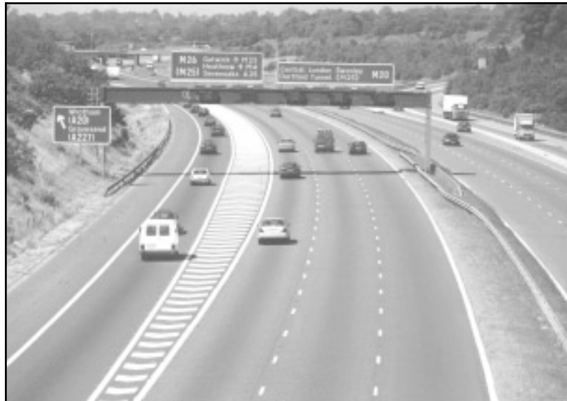
Tiger rail pavement markings on entrance ramp to freeway in England. Reprinted, with permission, from the Highway Agency, UK
