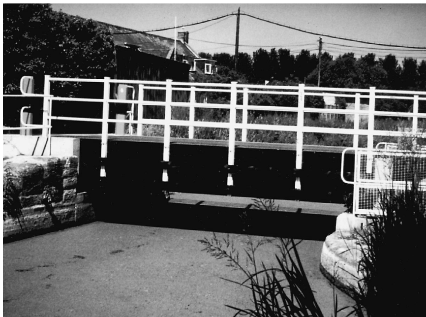
Figure 15. The Bonds Mill Bridge.
