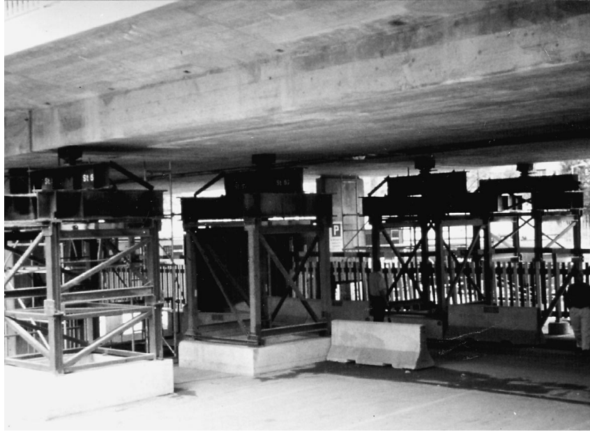
Figure 6. The Europa Bridge in Zurich.
