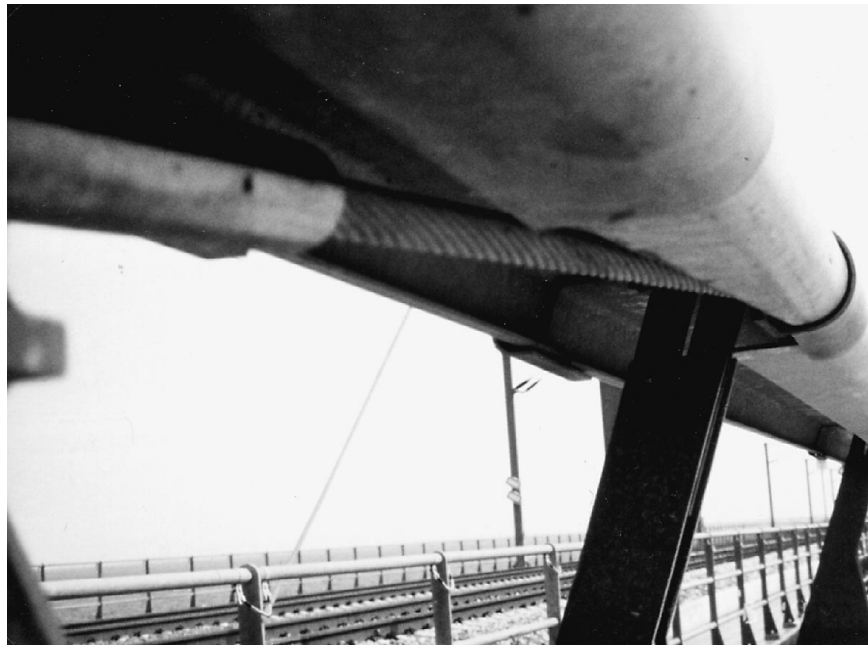
Figure 21. Bridge railing on the Great Belt West project.
