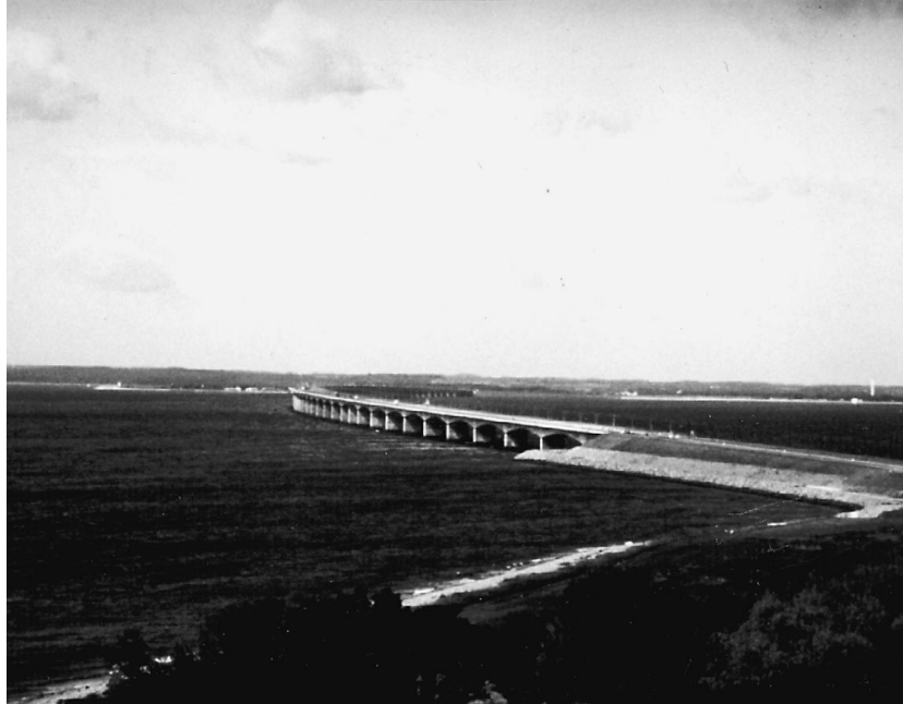
Figure 2. Great Belt Western Channel low bridge.
