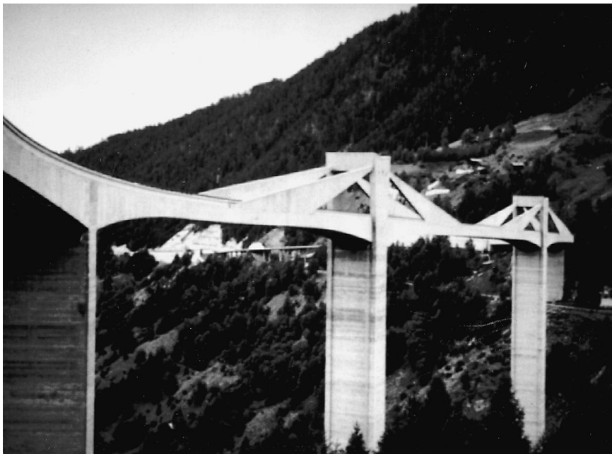
Figure 13. The Ganter Bridge at Simplon Pass.
