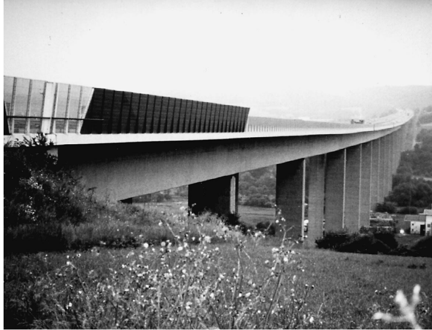
Figure 4. The Ahrtal Bridge.
