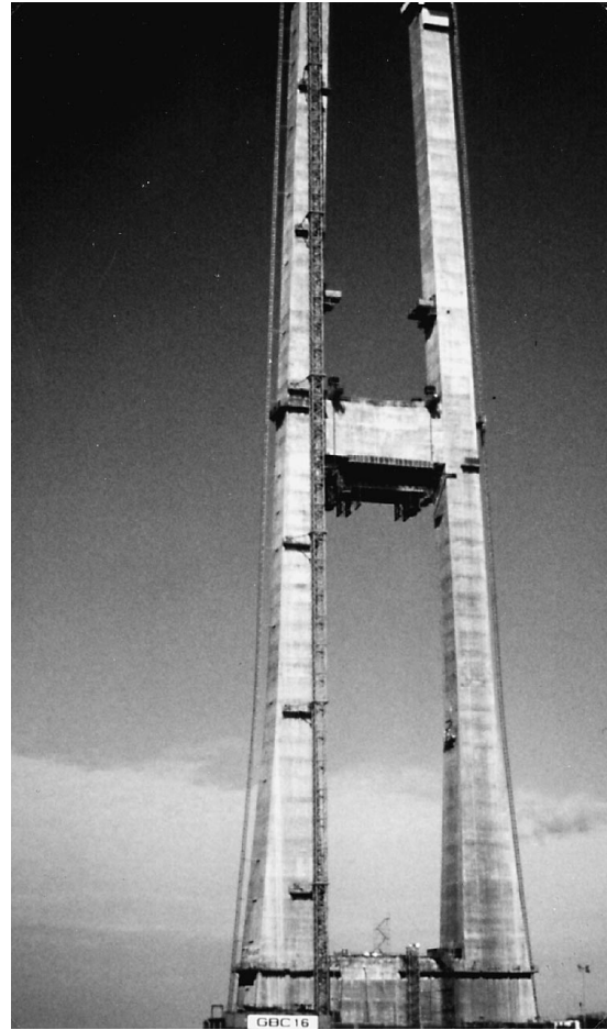
Figure 1. Great Belt Eastern Channel suspension bridge pylon.
