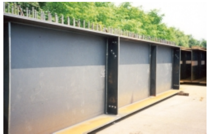
Figure 17. Fabricated components at Cimolai factory.
