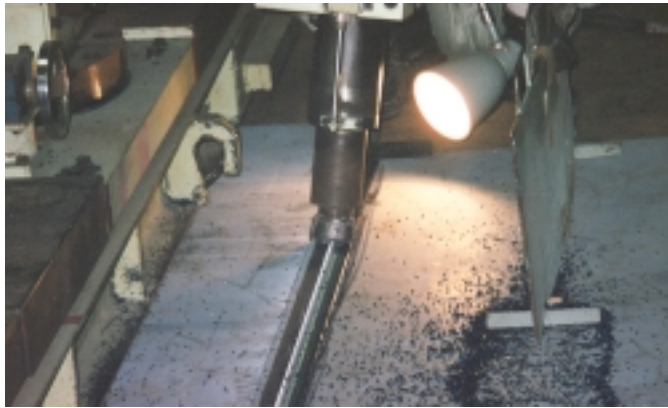
Figure 2. Double-bevel groove welds with root grinding machine at Sakai plant.
