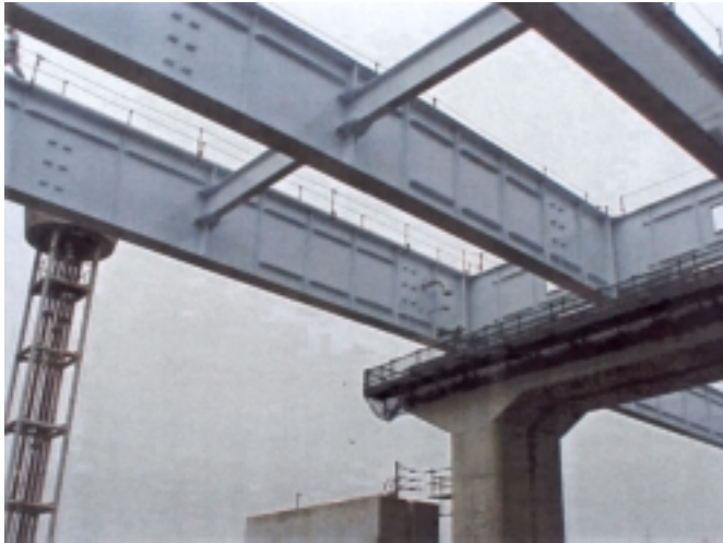
Figure 44. Shallow cross-beam diaphragms observed in Japan.
