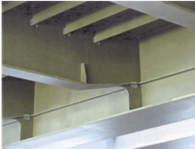
Figure 36. Floor beam field welds in German railroad bridge.
