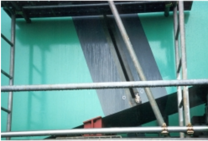
Figure 6. Preassembly of North Kyushu Airport Connection Bridge.
