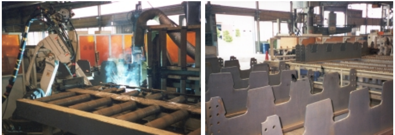
Figure 10. Transverse (orthotropic deck) rib assembly line at Tsu Works.
