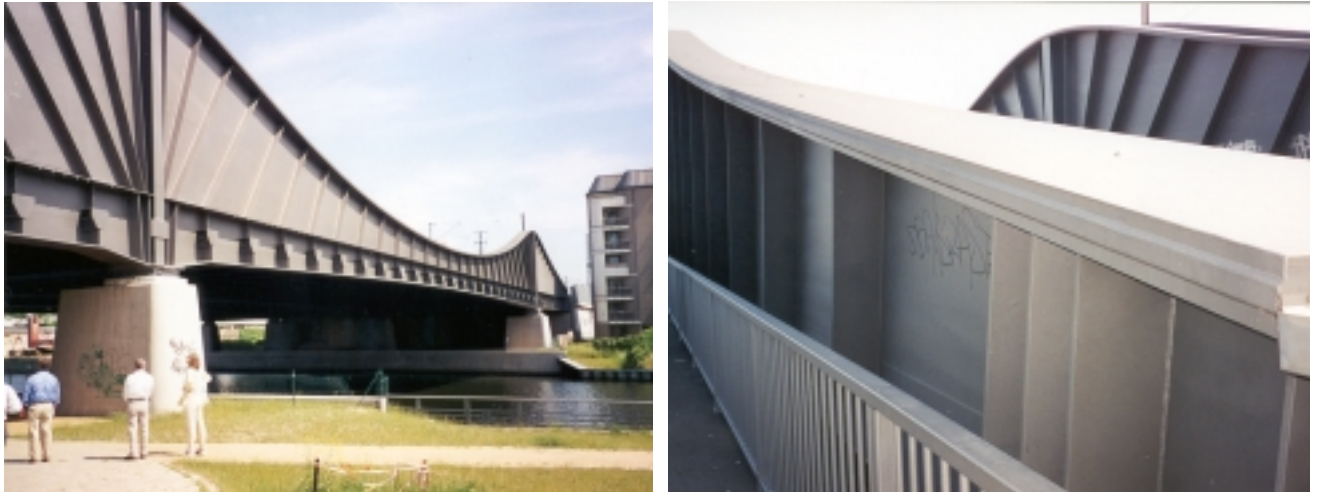
Figure 21. Havel River Bridge in Germany, fabricated from three 50-mm plates in a layer, was preassembled on site.
