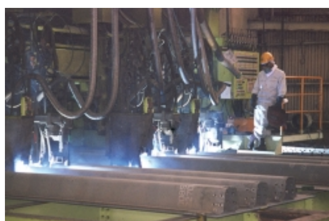
Figure 14. 20-electrode GMAW welding machine for open and closed rib welding to orthotropic deck plates at Shikoku plant.
