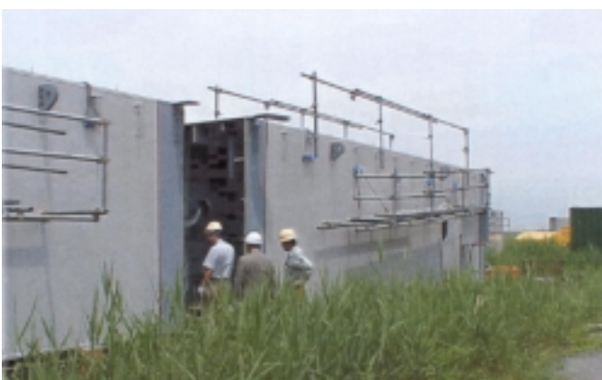
Figure 35. Welding of complete box sections together in the field in Japan.
