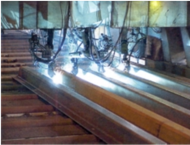
Figure 33. Automated multiple robots at NKK in Japan.
