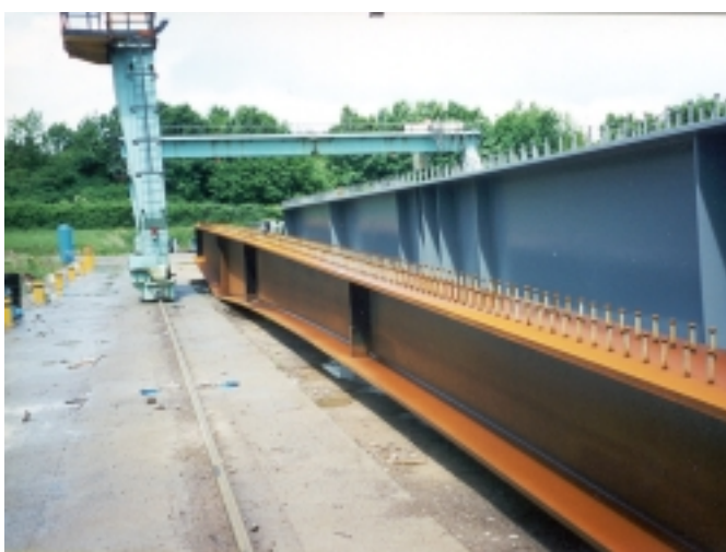
Figure 24. Fabricated components at Chepstow plant.
