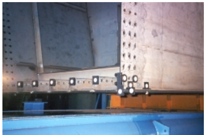
Figure 5. Box unit is measured for virtual erection check at Yokogawa plant.
