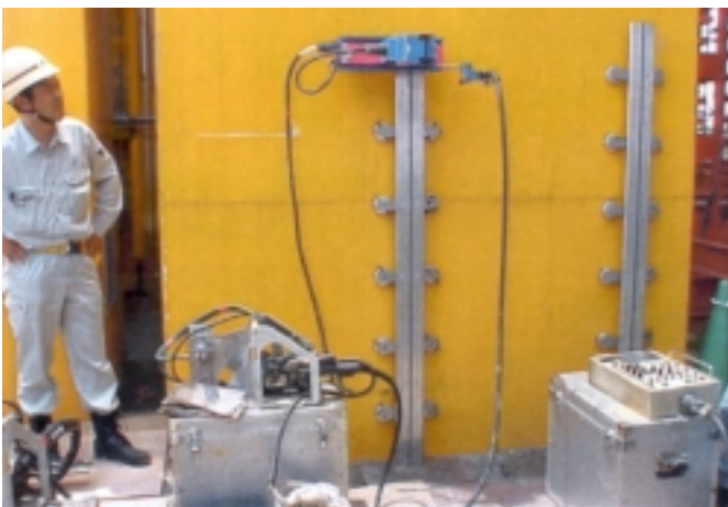
Figure 34. Automated GMAW vertical web welding setup in Japan.
