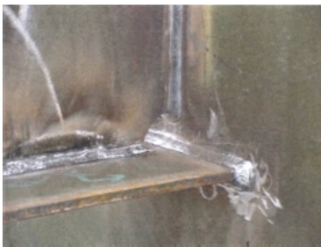
Figure 40. Wrapping of welds at cope at Kawada Industries in Japan.
