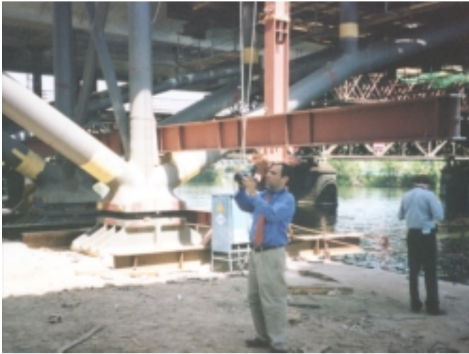
Figure 43. Unique cast joints at a railroad station in Berlin.
