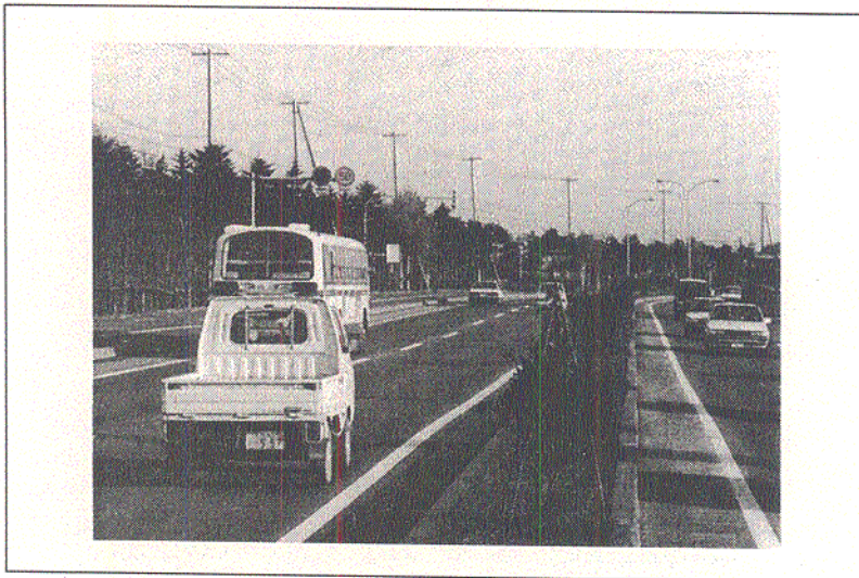
1. Ordinary National Highway Number 12, Iwamizawa City, Okayama. Highway snowbreak forest. (Hokkaido Development Department)
