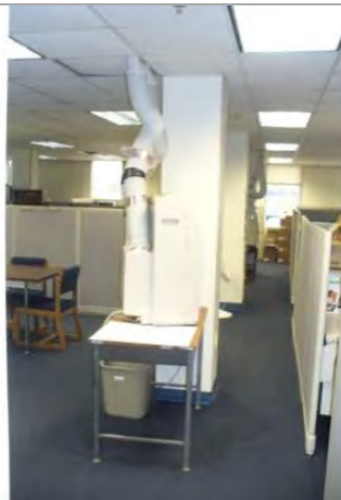
Figure 13.-Building 1 has portable dehumidifiers due to inability of building HVAC systems to handle high humidity in the building.
