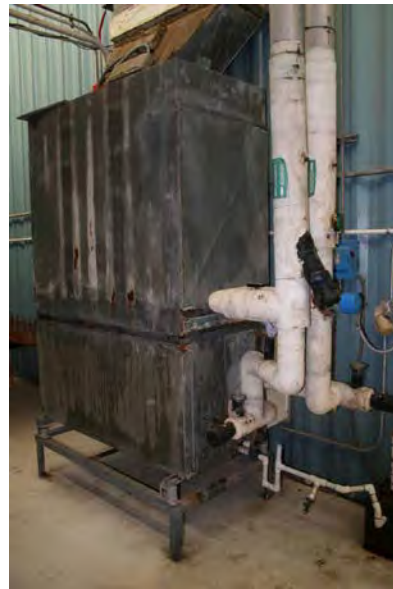
Figure 3.-Replace Chilled Water Air Handling Unit
