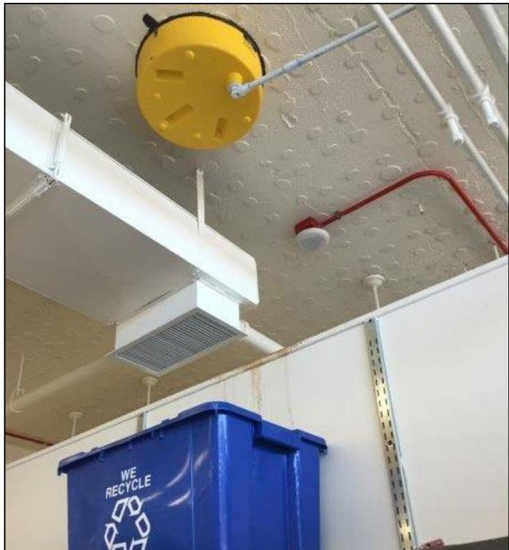
Figure 5. Catchment system to drain roof leaks in Spanagel Hall electronics lab spaces.
