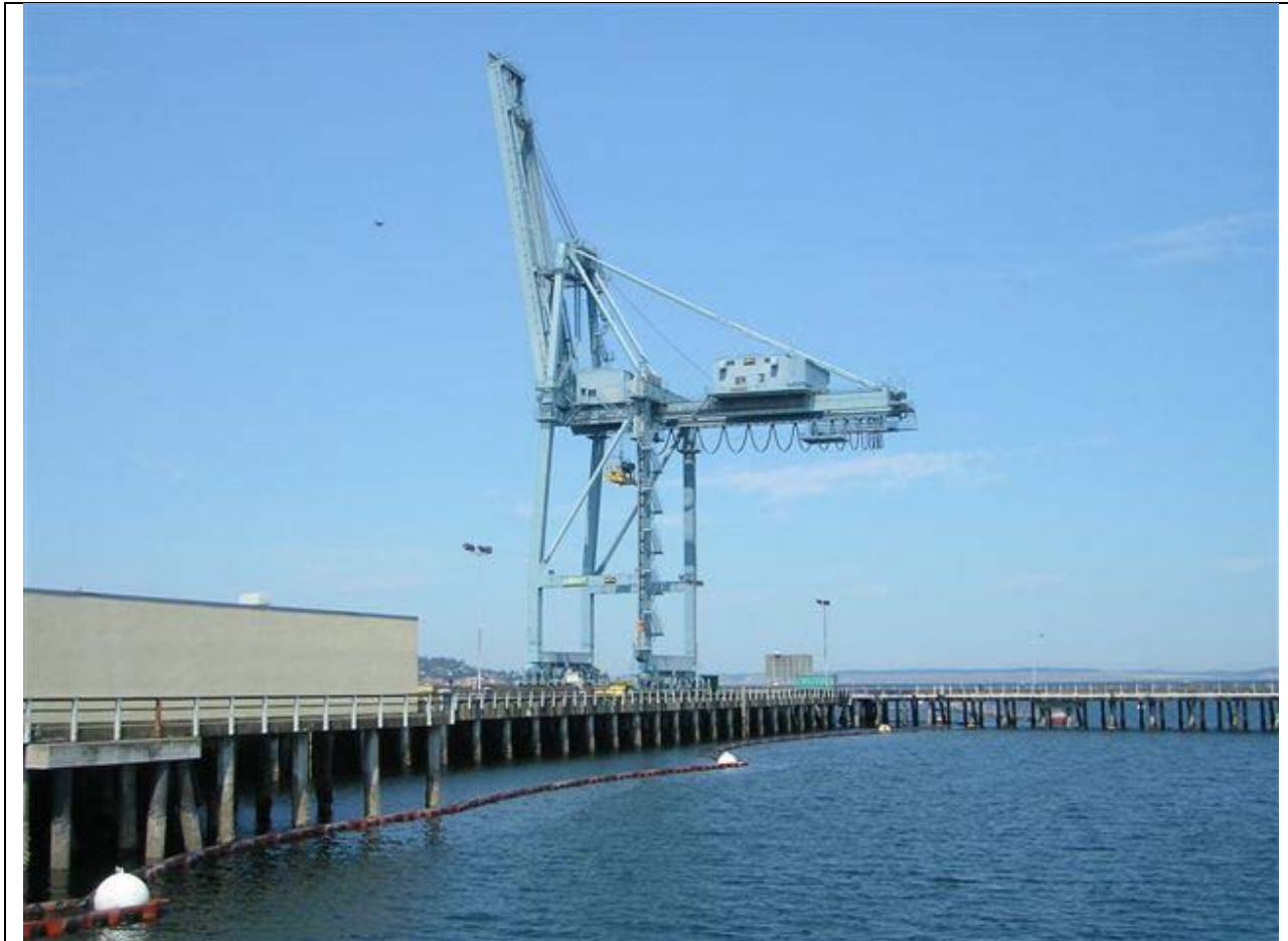
Figure 1. "Big Blue" Container Crane at Naval Magazine Indian Island.
