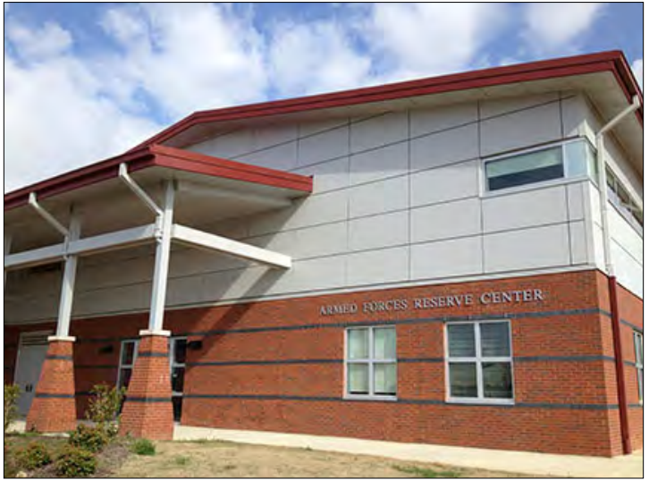
The Alabama National Guard opened a new Armed Forces Readiness Center on December 18, 2013 at the Alabama National Guard base in Birmingham, Ala. The new AFRC has been awarded the U.S. Green Building Council's Leadership in Energy and Environmental Design (LEED) Gold certification
