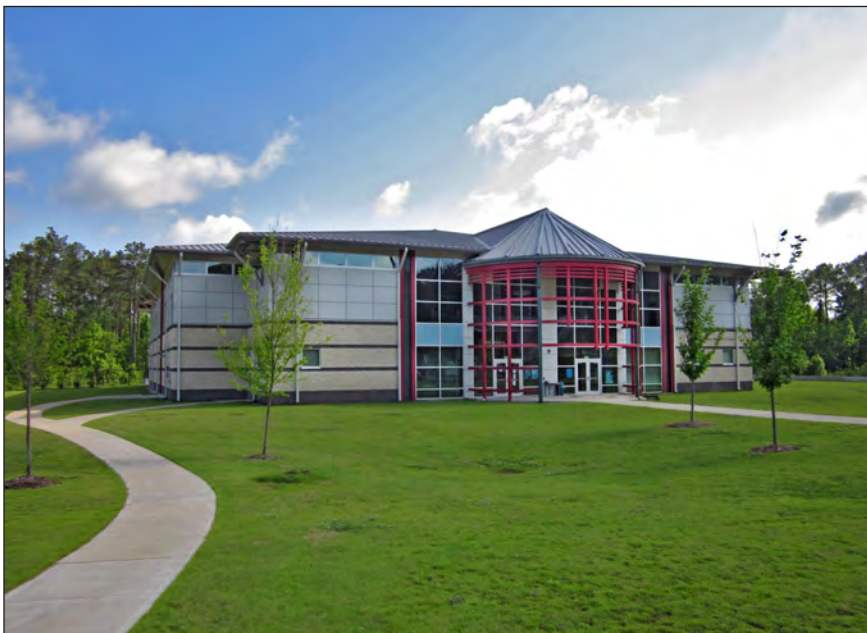
To minimize our impact on the environment, as well as save taxpayers' money, the Alabama Guard is proud to open the first LEED Platinum certified commercial building in the state of Alabama. The new Armed Forces Reserve Center is located on Pelham Range in Alexandria, Ala. (Photo by Dean Sharp, JMR Architecture, PC)
