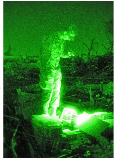
Day and night, Soldiers worked in the aftermath of the April 27 tornadoes. (Photo by Spc. Brenda Thomas, Public Affairs Office)
