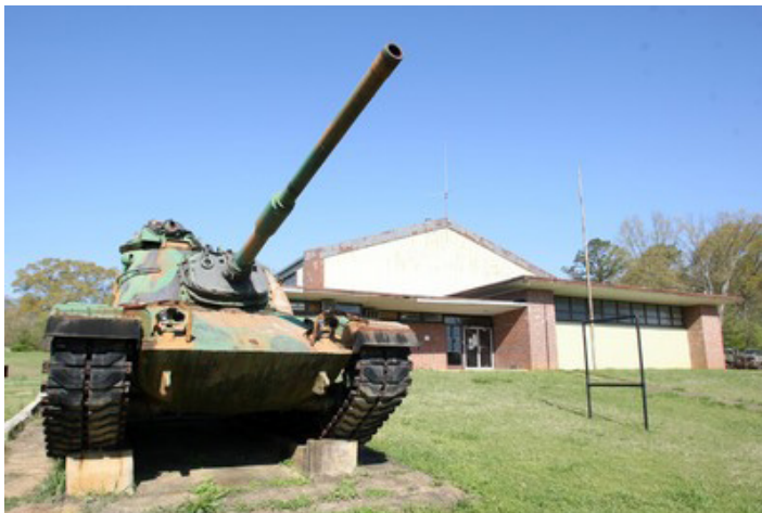
The armory in Heflin, Ala., is one of thirteen armories in Alabama scheduled to be closed by the end of fiscal year 2012. (Photo from The Anniston Star , used with permission)
