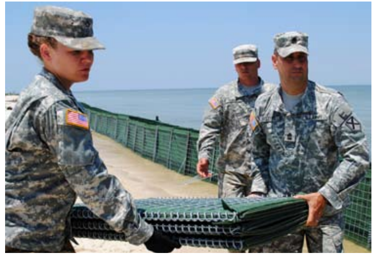
Soldiers from the 62nd Troop Command erect HESCO barriers on Dauphin Island during the Deepwater Horizon disaster response.
