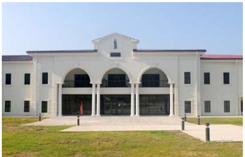
This Armed Forces Readiness Center at Fort McClellan is home to the 167th TSC
