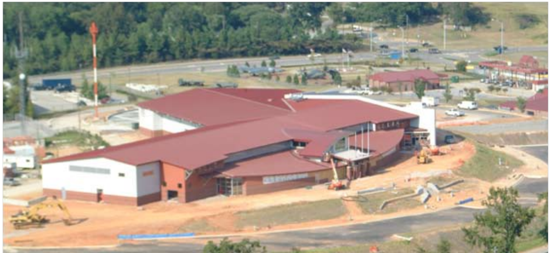
New armory under construction in Birmingham
