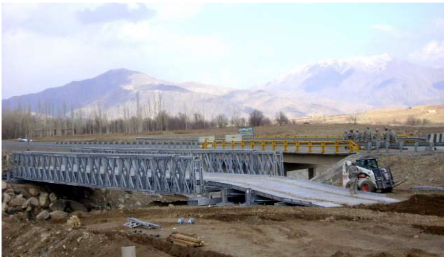
Alabama National Guard Engineer Soldiers building a bridge in Afghanistan
