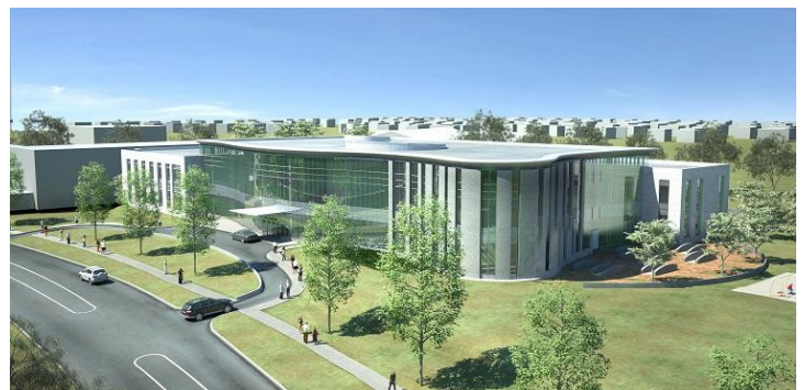
Artist’s Rendition of the NICoE currently under construction at NNMC
