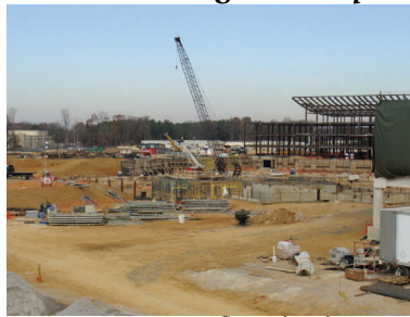
Basement of Building C
