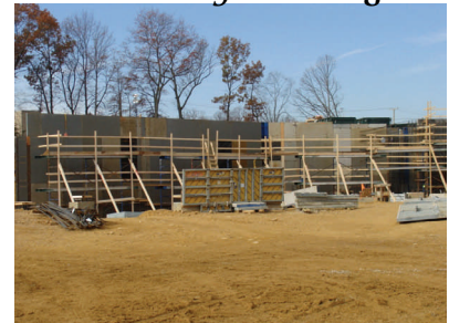
1st Wall Pour of Building C
