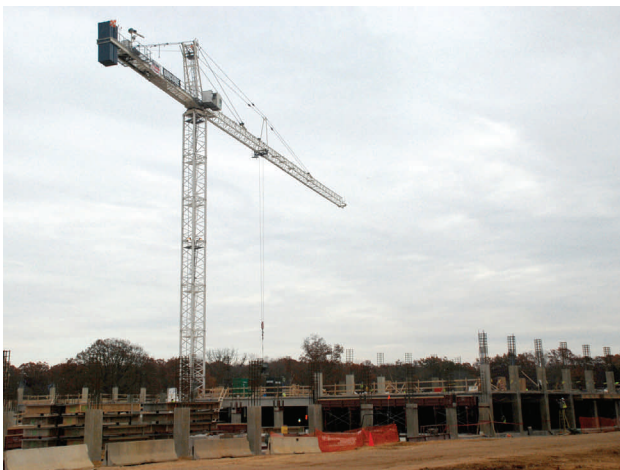
North Parking Garage
