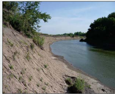
River Bank Erosion
