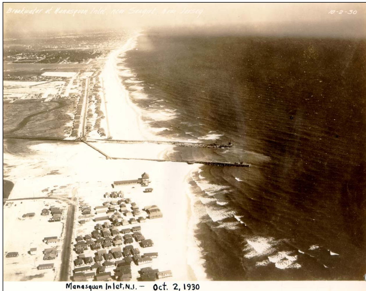
Figure 7. Construction of Manasquan Inlet jetties, New Jersey, October 2, 1930, view looking north. Material for the jetties was supplied via an elevated roadway that extended out to sea from the land. Note that sand is already accumulating on the south (lower) side of the south jetty. The shoreline is continuous, and at this site the inlet was dredged after the jetties were completed.
