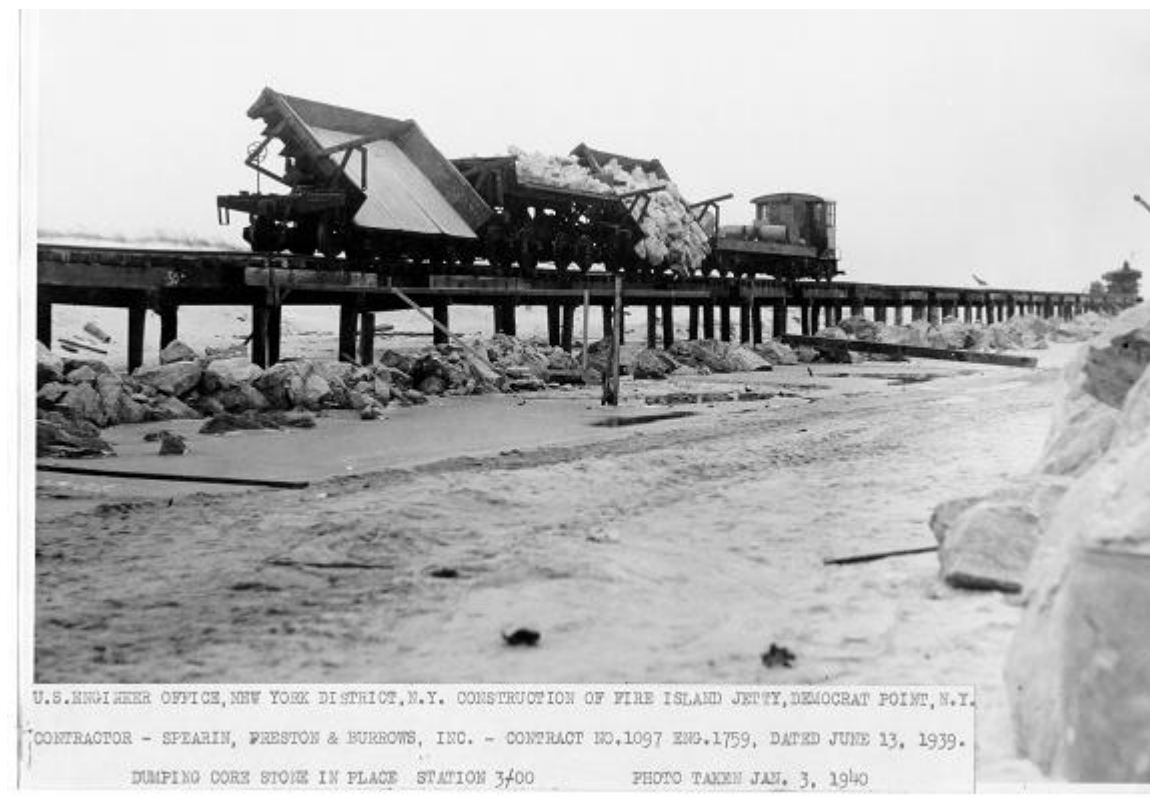
Figure 6. Construction of the Fire Island jetty on Democrat Point, at the west end of Fire Island, Long Island, New York, January 3, 1940. Many early USACE jetties were built from the land moving seaward using materials brought in by train.
