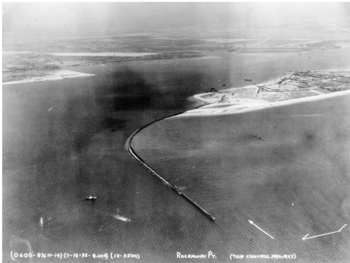
Figure 5. Construction of the jetty on the east side of Rockaway Inlet, Long Island, New York, July 12, 1932. The urban area on the opposite side of the inlet is the east end of Coney Island, and Jamaica Bay is in the distance. In 7 decades, the fillet has filled with sand to approximately the end of the jetty seen in this image.
