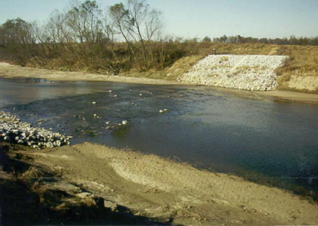
Grade control sills, immediately after construction
