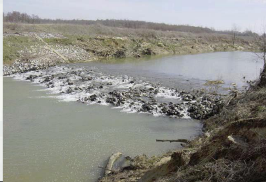
Grade control sills, after 10 years
