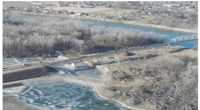
Figure 2. Bridge Abutment Repair at Decatur Bridge
