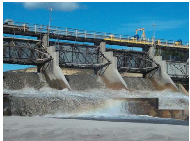
Figure 2: Sediment laden water flowing over the main gates early in the Spencer Dam flush.
