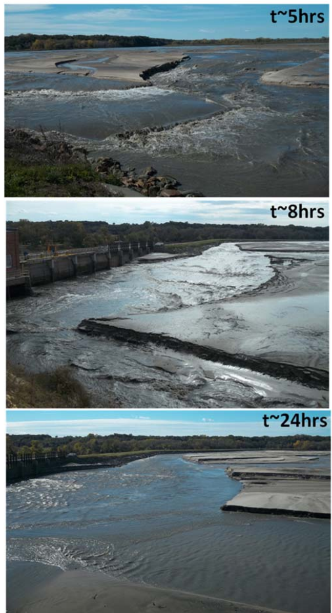
Figure 3. Evolution of the Spencer Reservoir sediment delta during the flush. The head cut propagated upstream shortly after the flushing gate was opened (top). Then the channel deepened and widened the rest of the first day (middle), until it settled into a form close to the final geometry 24 hours after the flush (bottom).
