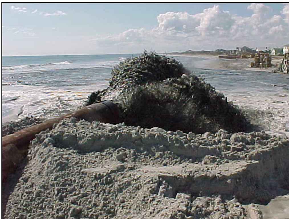
Figure 1. Dredging at St. Augustine Inlet, Florida
