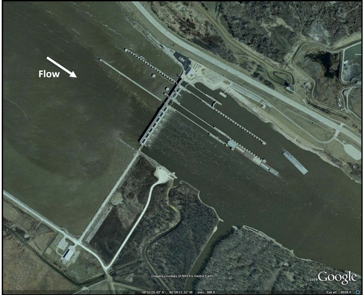
Figure 2 - Aerial photograph of Mel Price Lock and Dam
