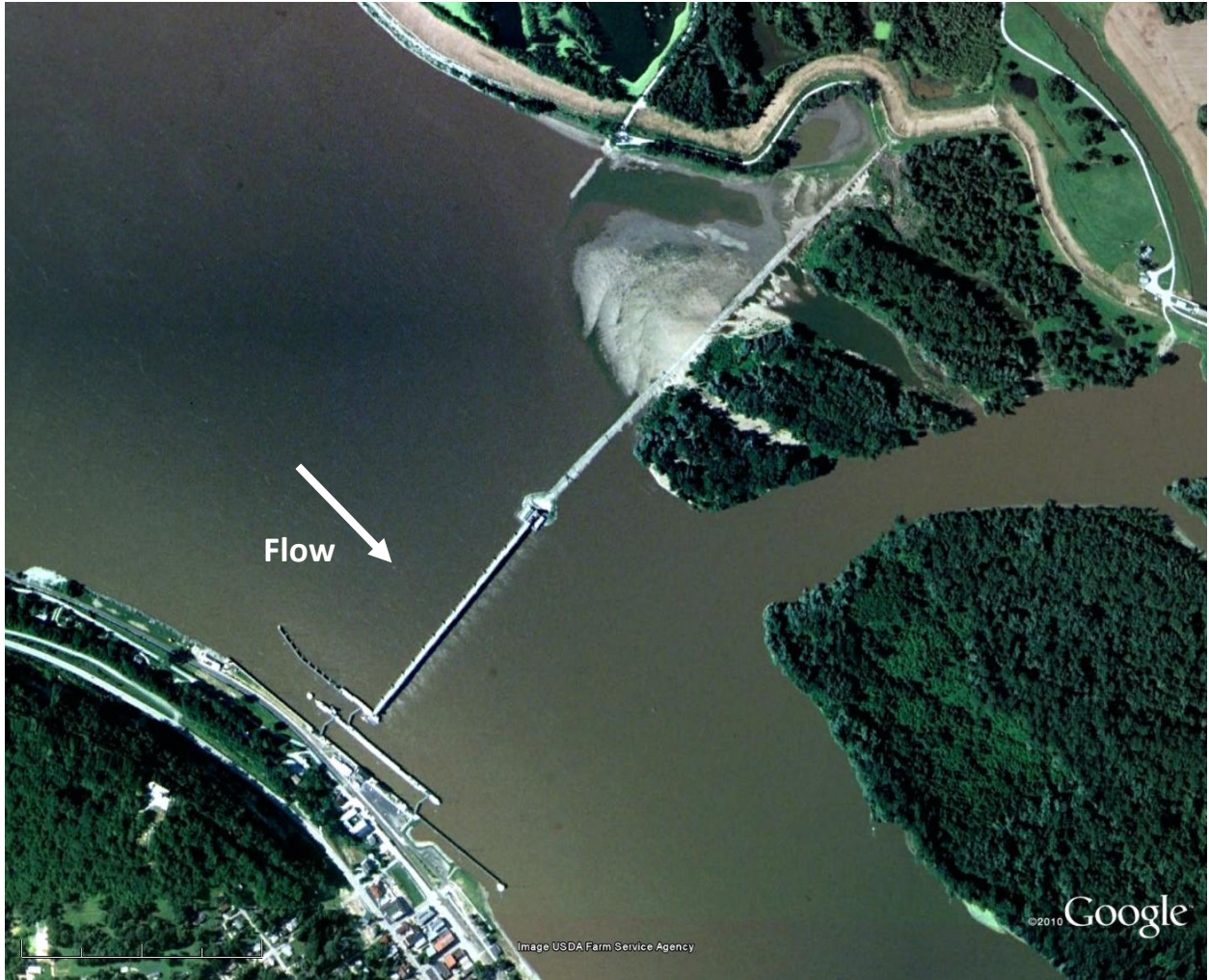
Figure 2 - Aerial photograph of Lock and Dam 24
