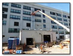
heating plant to natural gas fired de-centralized heating systems. The conversion to natural gas started in FY13 with a Corps of Engineers project to convert buildings 112, 144, 145, 154, and a portion of 299 to natural gas. In FY14, JMTC started the conversion of 10 factory buildings (208,
