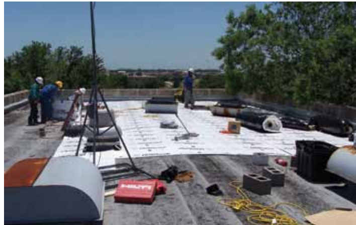
Workers finish the roof of a “green” building under construction at Fort Hood, Texas. The building is designed to meet the U.S. Green Building Council’s Leadership in Energy and Environmental Design (LEED®) silver-level criteria.
