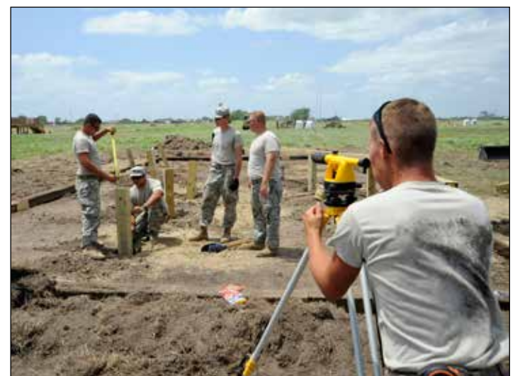
Just Right: Soldiers assigned to the 623rd Engineer Company work together to level and align posts needed for one of the obstacles being built for a new course at Greenlief Training Site near Hastings, Neb. The Soldiers built the obstacle course as part of the company's 2016 two-week annual training.
