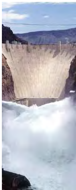
Hoover Dam on the Colorado River, is a feature of the Boulder Canyon Project (Managed by the Reclamation Project in partnership with USACE). Located on the Arizona-Nevada state line, at 726 feet it is the highest concrete dam in the United States, a National Historic Landmark, and one of America's Seven Modern Civil Engineering Wonders. Photo from: http://www.usbr.gov/lc/hoover-dam/gallery/damviews.html .
