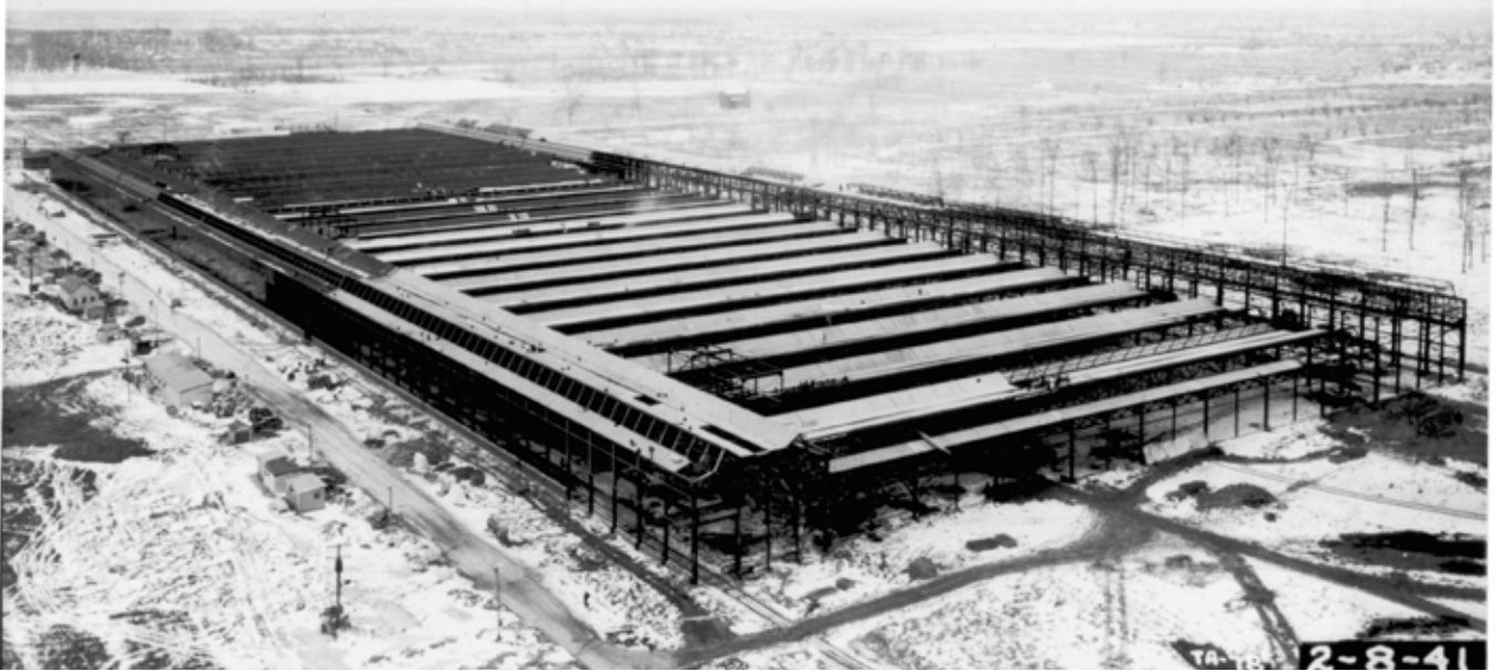
The nearly completed Detroit Arsenal Tank Plant in 1941.
