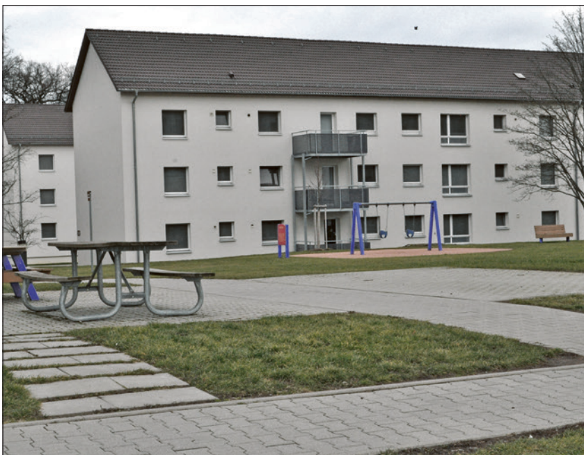
The 1,300 family housing units available in USAG Stuttgart are stairwell apartments with two to five bedrooms that are spread throughout four of the five installations (there are no housing units on Stuttgart Army Airfield).
