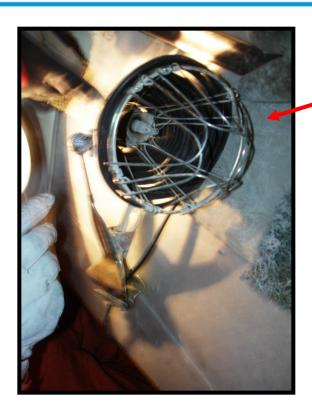
Example of temporary light fixture with clamp that was used inside containment area.
