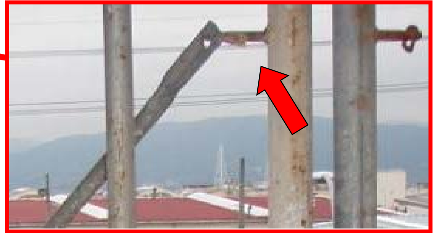
Unsecured "X" bracing at the point of the fall.
