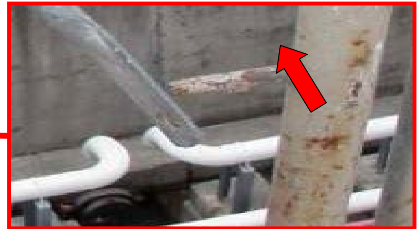
Unsecured "X" bracing at the point of the fall.
