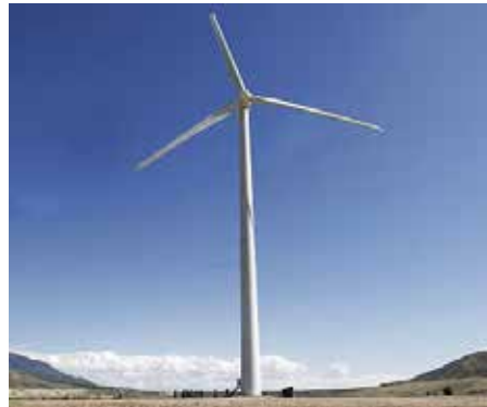
1.5 MW Wind Turbine Tooele Army Depot
