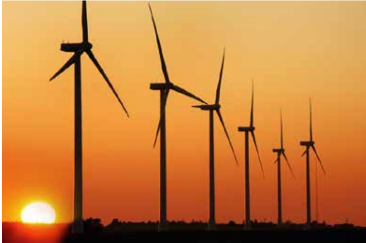
Photo from Alstom 2010, NREL/PIX 18207
