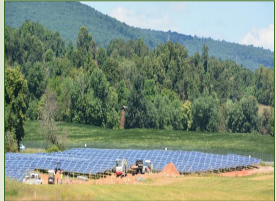
Ongoing construction/installation of solar panels at Fort Detrick, Maryland
