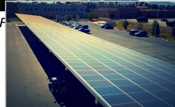
Reserve Center, Arizona
