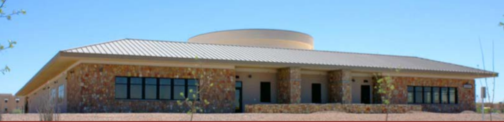
Fort Bliss power plant. Photo from FEMP, NREL 17255
