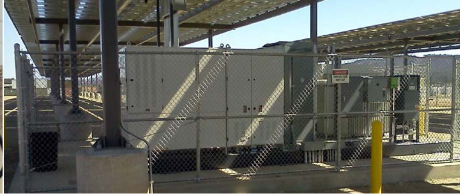
Figure 35. Power Electronics for the Phase 2 Solar Array. Photo by Lars Lisell, NREL
