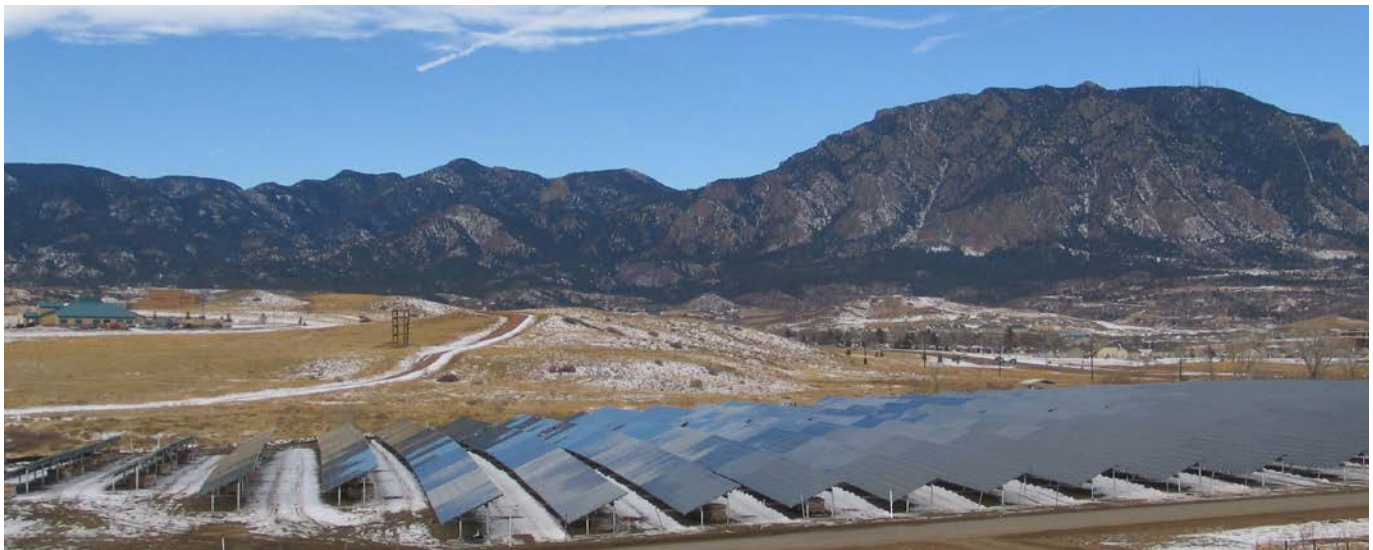
Figure 20. Fort Carson solar array. Photo from Fort Carson
