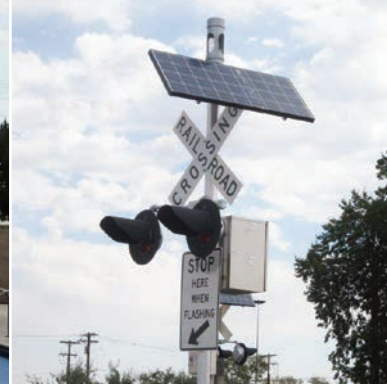
Figure 49. Solar railroad crossing lights. Photo from Sierra Army Depot
