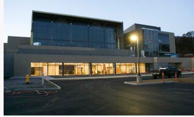
Figure 43. The Dalles Readiness Center under construction Photo from U.S. Army
