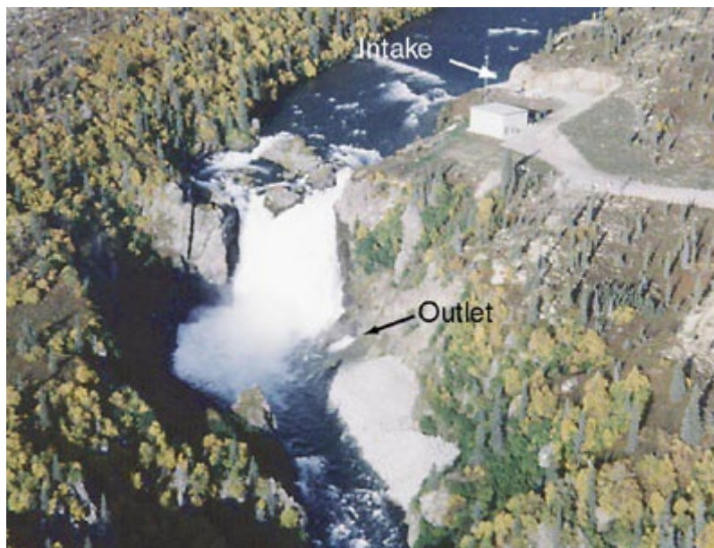
Figure 23. Diversion hydropower plant. 89
