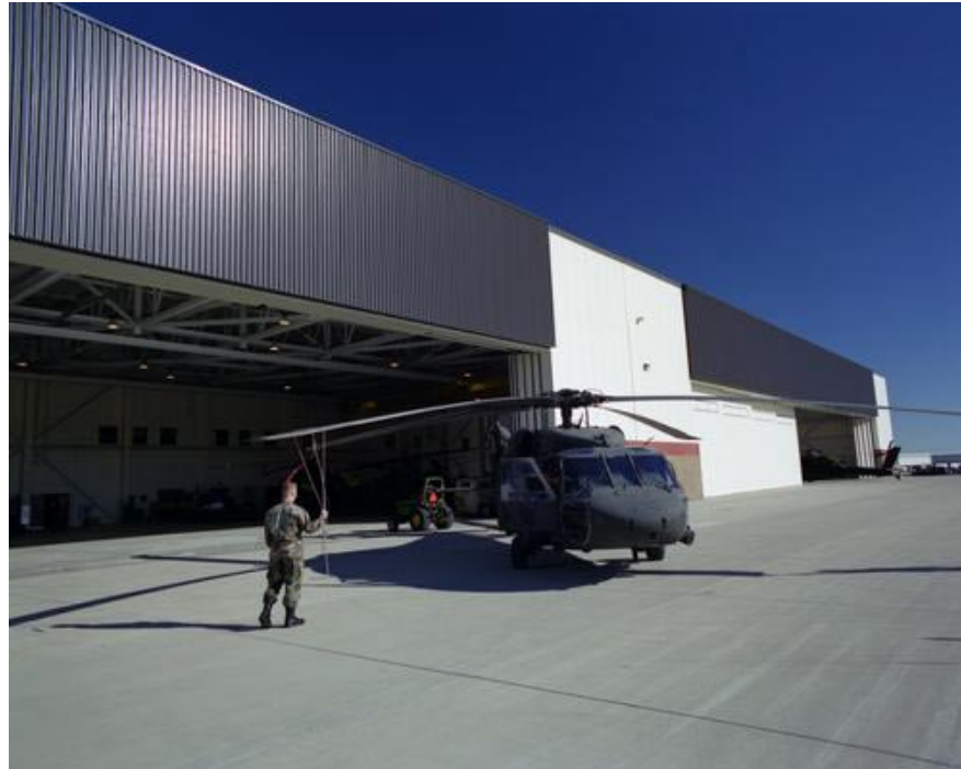
Figure 90. Fort Carson solar walls. 171
