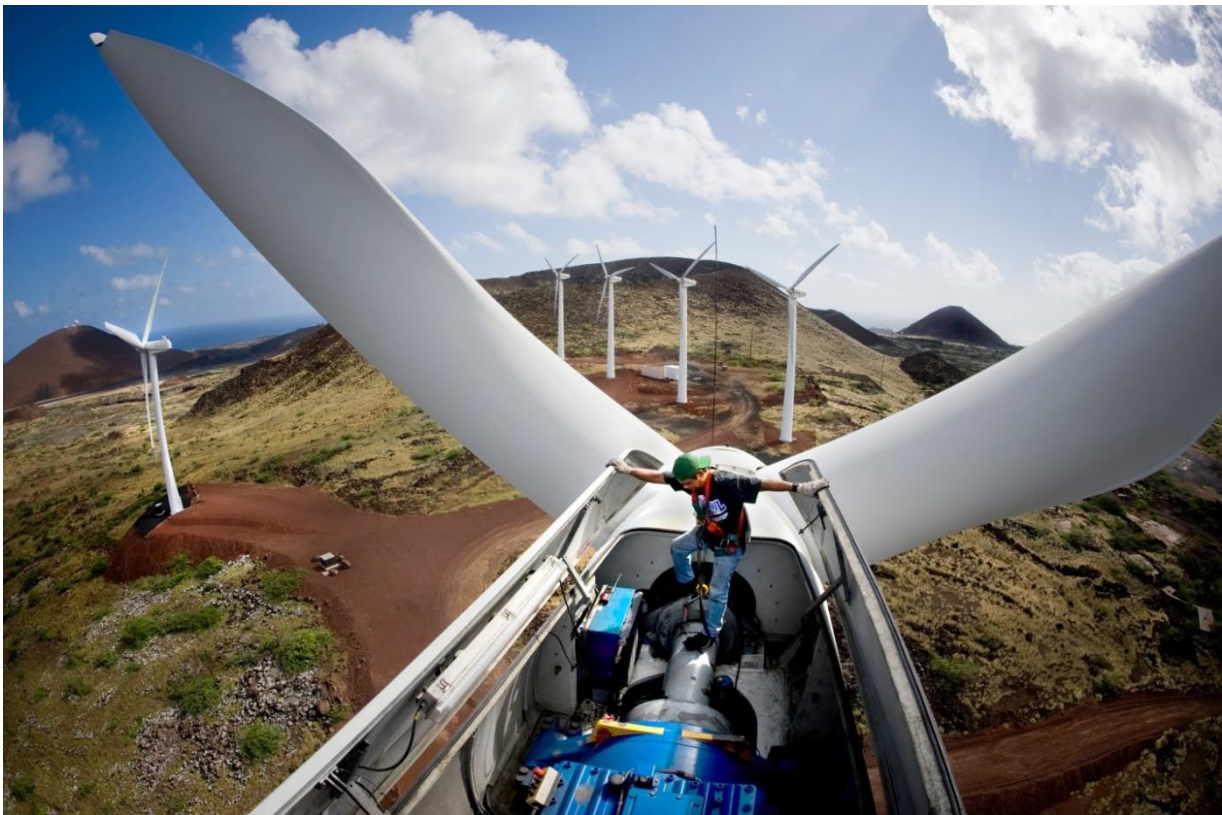
Figure 108. Performing maintenance at wind farm on Ascension Island. 213
