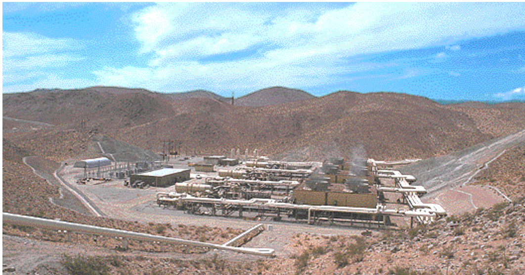
Figure 164. The geothermal power plant at China Lake. 308
