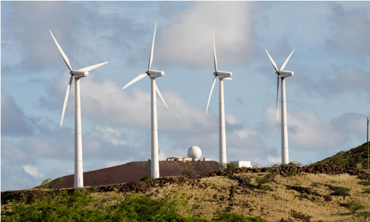
Figure 92. Four of six wind turbines in operation at Ascension Auxiliary Airfield. 174
