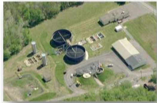
Tobyhanna Army Depot Wastewater Treatment Plant
