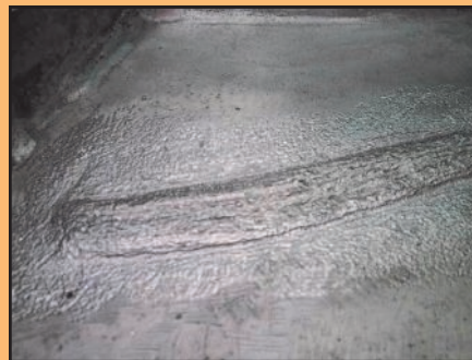
Localized crack repair treated with UIT.
